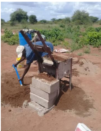
Making the bricks on site
