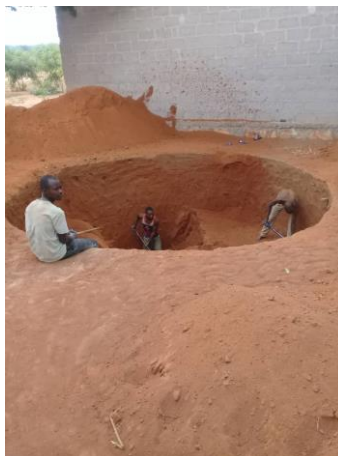
Digging tank construction
